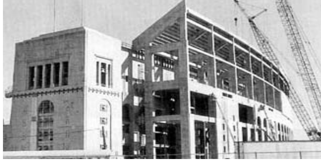
“Shoe” addition construction 1999-2000
