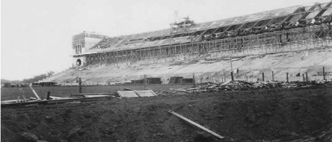
The Ohio State University Football Stadium under construction
